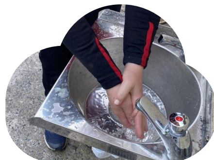
Outdoor hand washing facilities.
